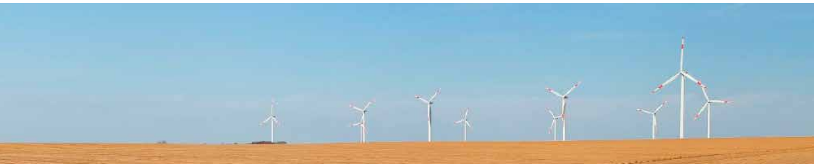
Windpark Titz 10 x 2,05 MW Repower MM92
